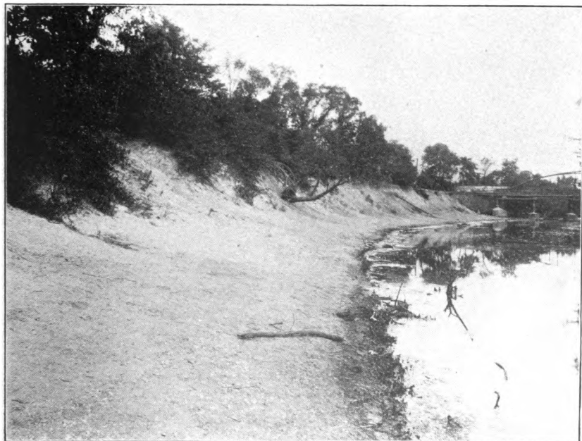
24. Eroded bank on the Desplaines River near Madison Street bridge.
