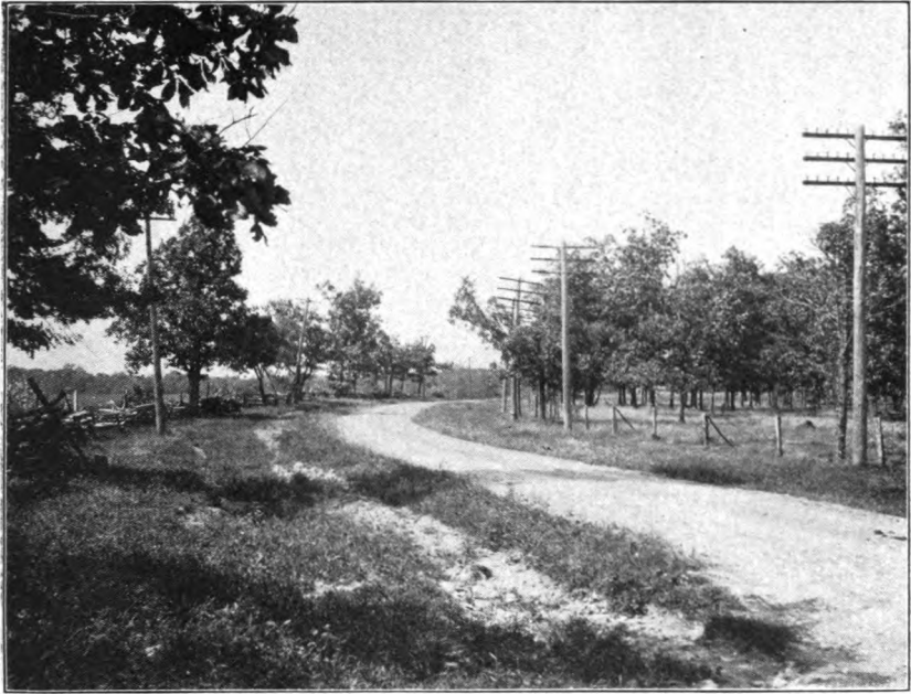
6. Green Bay Road in Glencoe, looking north.
